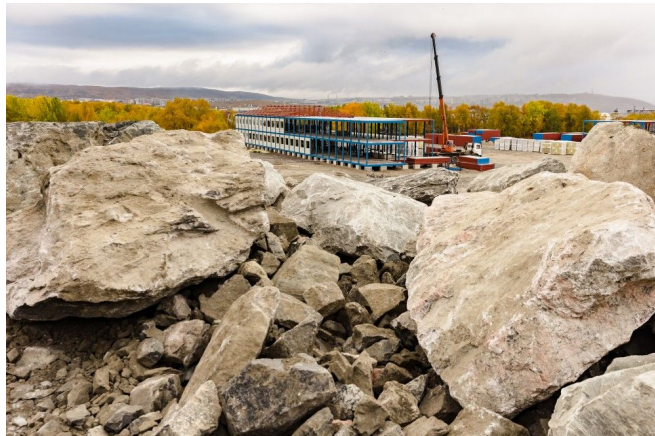
First, the camp for workers is to be built. Then, construction of the port facilities by the Kola Bay will start. (Ministry of Information Policy of the Murmansk Region via The Independent Barents Observer)
